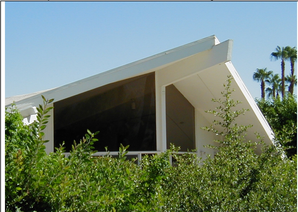
P5b. Description/Date of Photo: View of south elevation, August 2002.
